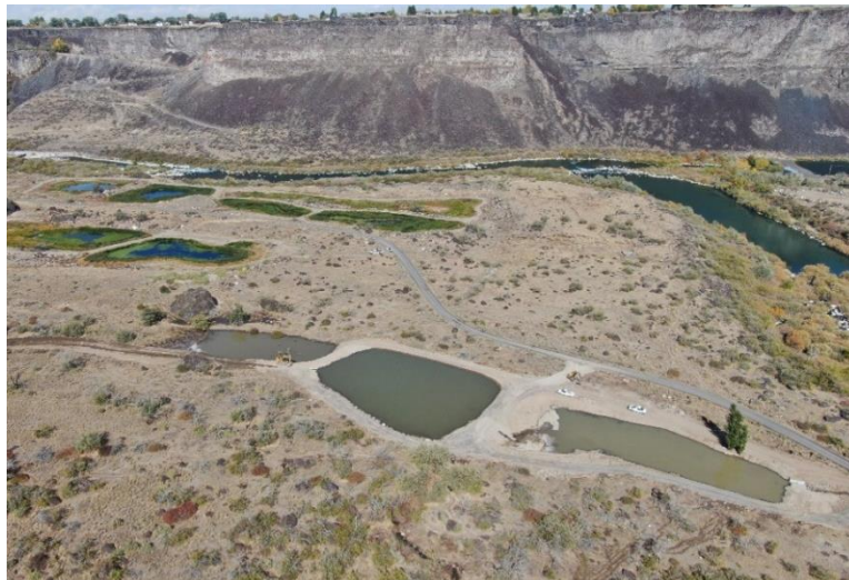
Auger Falls Water Quality Ponds
