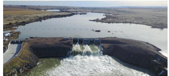
Service Spillway in Operation (March 21, 2017)
